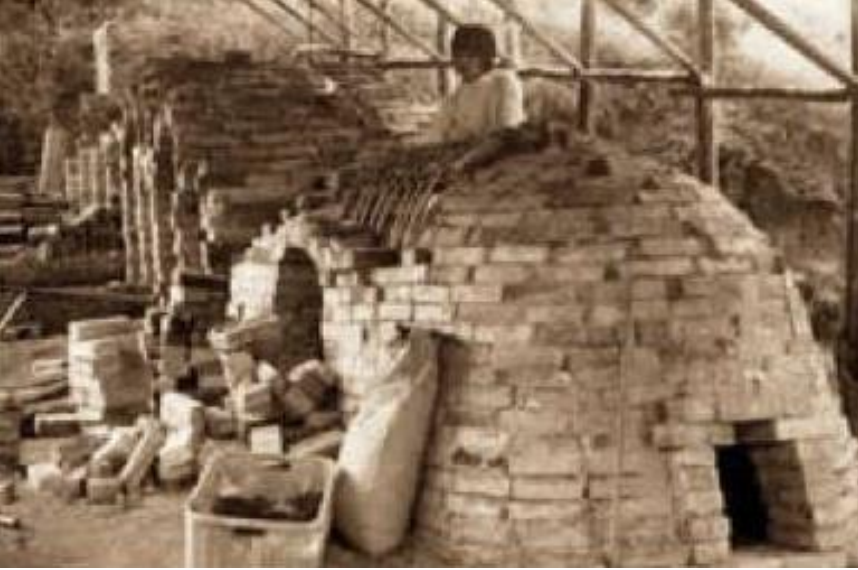
Top: Building the first noborigama . Ateliê do Antigo Matadouro, 1975, Cunha. Bottom left: Kiln opening after the first collaborative firing Cunha, 1976. Bottom right: Old Slaughterhouse before transformed into a collective potter's studio, 1975. Photos from Alberto Cidraes personal archive
